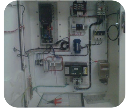
L Shaped subpanel with Allen-Bradley® Drive installed. Enclosure shown with cooling unit mounted to right side.
